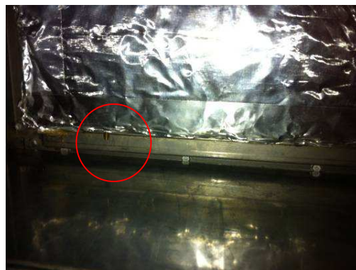
Barbed Fitting shown circled above (located on bottom of flue collection box, below induced draft blowers)
