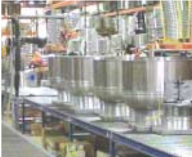
View of plant from the turret punch's auto sheet loader
