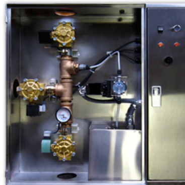
PCU CORE Control Panel
