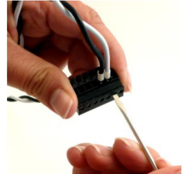
Figure 11 – Current Transformer Wiring
