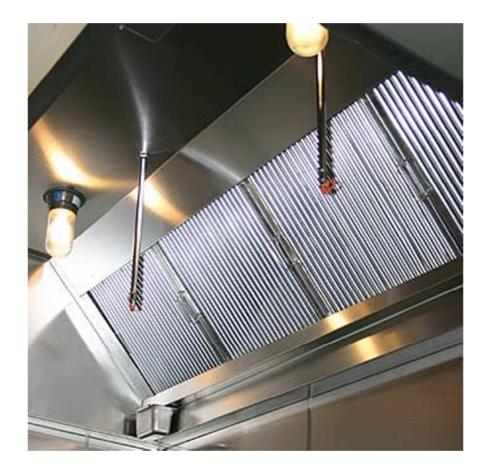
ALL FILTERS ARE TESTED TO THE ASTM F2519-05 GREASE PARTICLE CAPTURE EFFICIENCY OF COMMERCIAL KITCHEN FILTERS AND EXTRACTORS.
