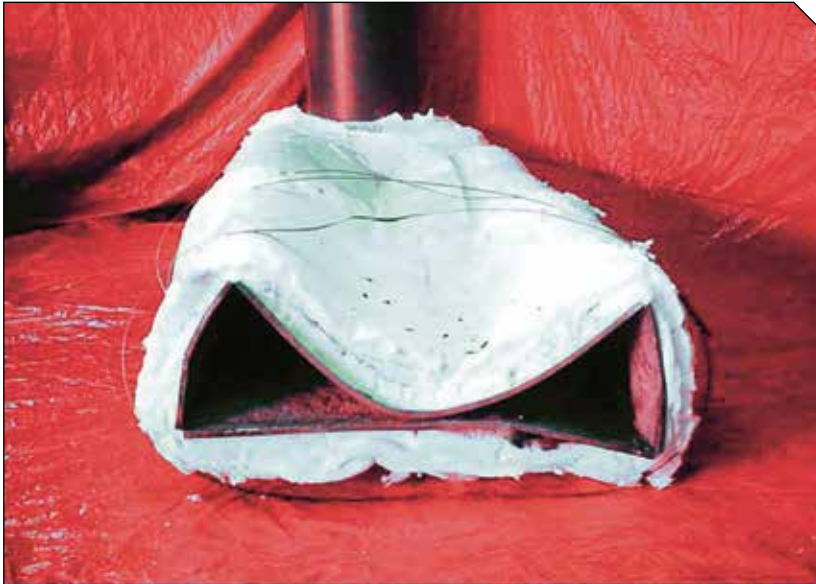
FIGURE 4. Collapsed unlisted duct after fire testing to listed duct standard UL 1978.
