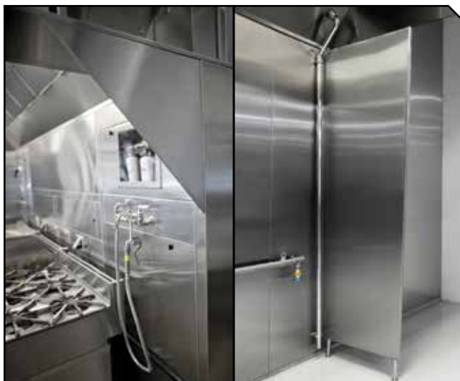
FIGURE 3. Photos of triangular quarter end panel and full end panel, tapered and double-wall insulated.
