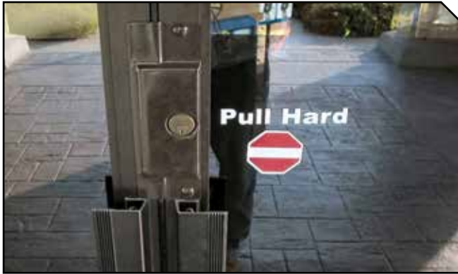
FIGURE 7. Consequence of negative air balance.
