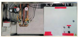
FIGURE 5: Electronic fire suppression system components in hood end utility cabinet.
