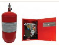
FIGURE 2: Wet chemical system release assembly cabinet and agent cylinder.
