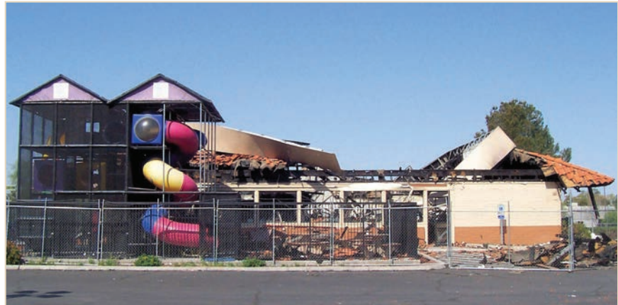
PHOTO 1 Total loss fire damage at quick service restaurant.
