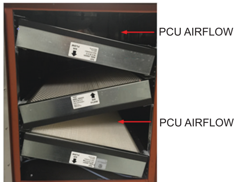
Figure 19 - Filter Installation
